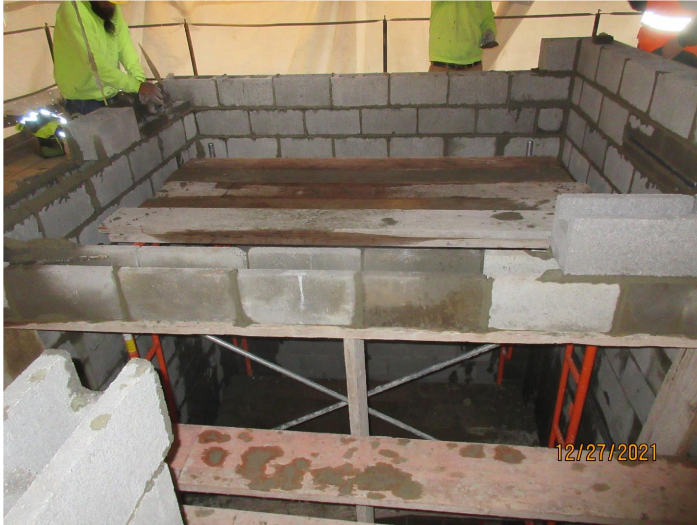
CMU Elevator Shaft at Building B
