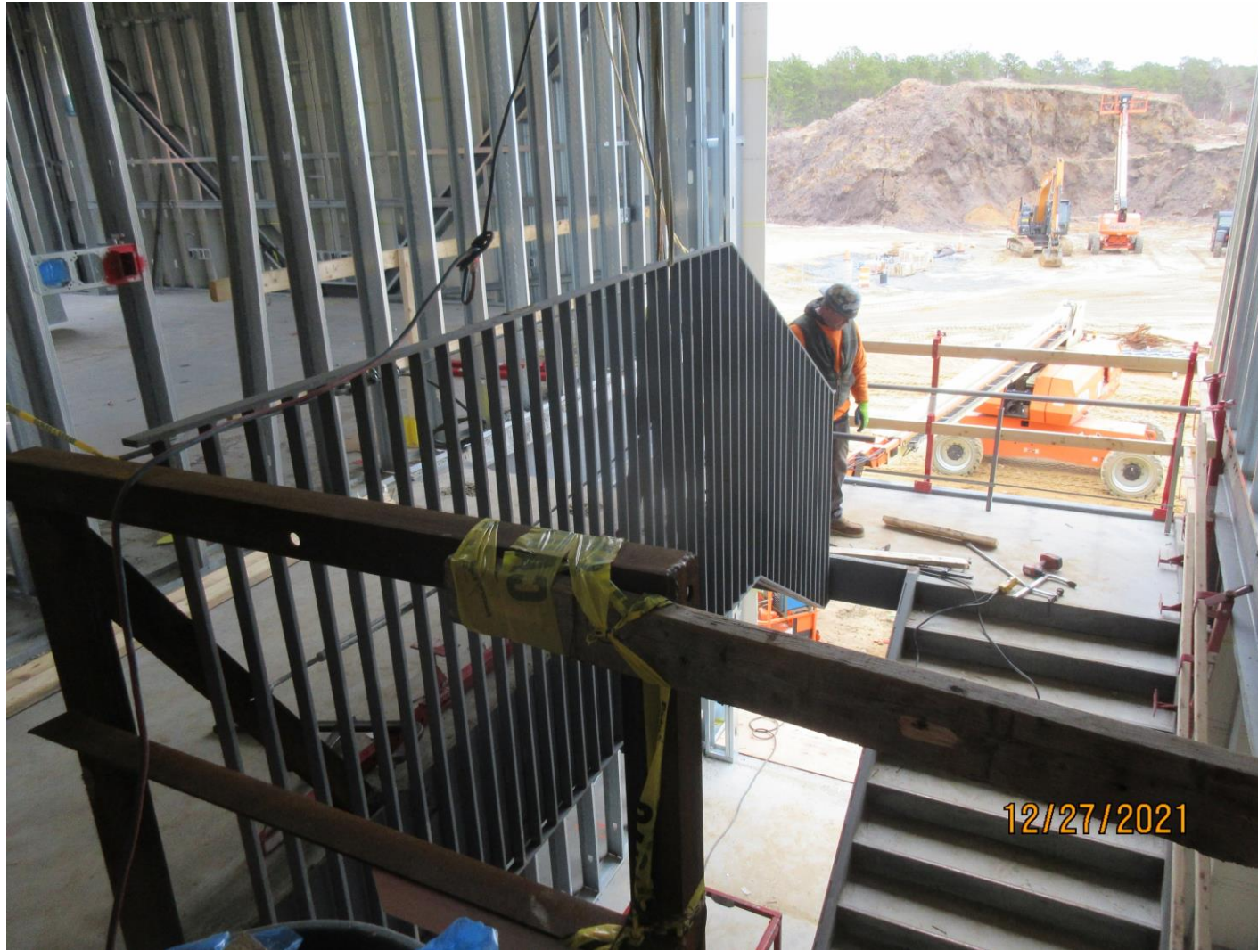
East Stair Rail Installation at Building D
